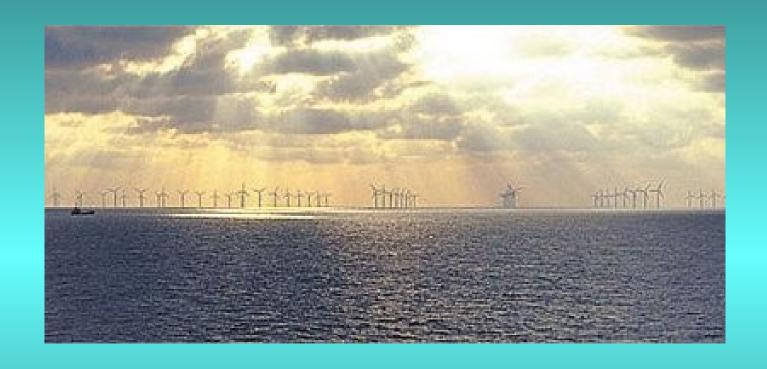
20 km from the coast of Denmark, you will find "Horns Rev", the biggest wind farm in the world. 80 turbines 110 m tall, capable of 160 MW
